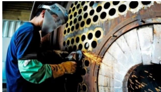
Gambar 6. Proses Perapihan Mesin Boiler
